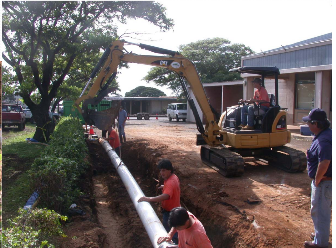
Replacement under Lyle's expert supervision
