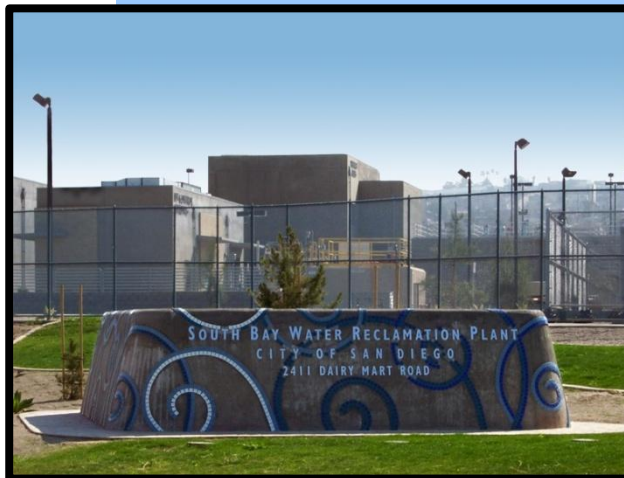
South Bay Water Reclamation Plant
