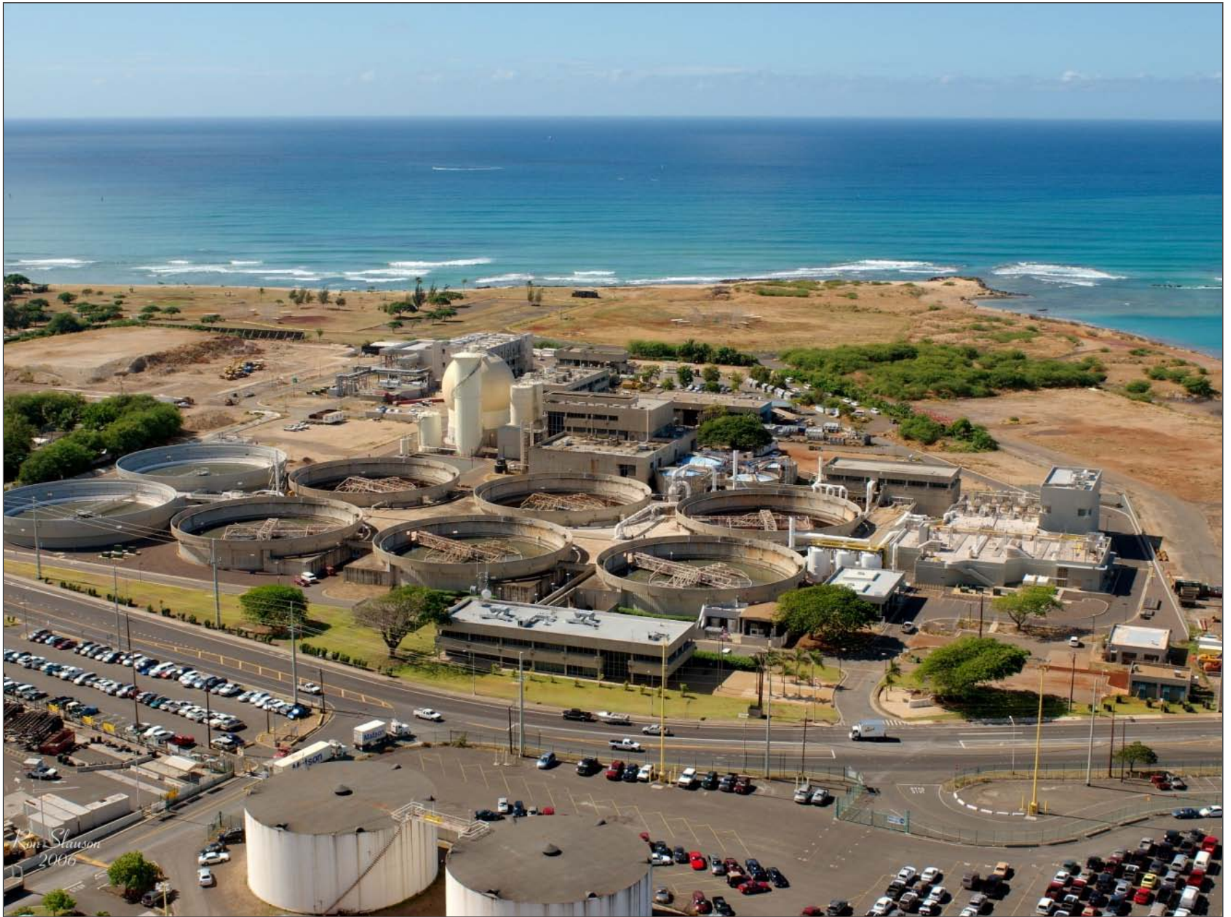
Sand Island WWTP – Sand Island State Recreation Area.
